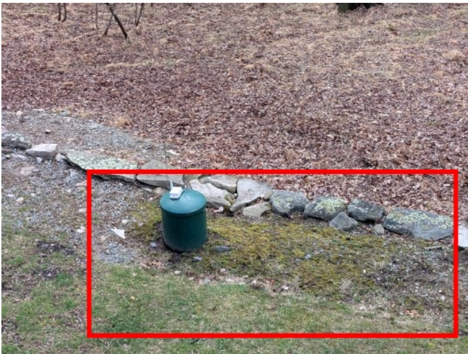
In Ground Propane Tank
