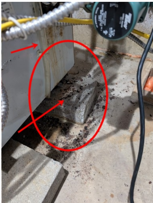
Rust staining and loose pieces
