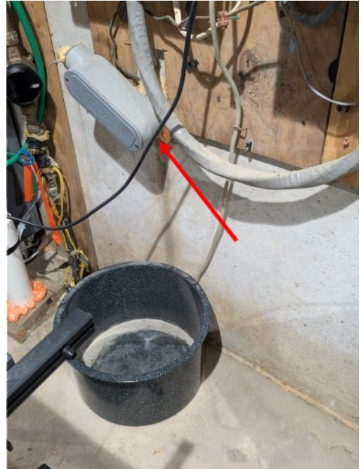
Indication of Prior Leak
