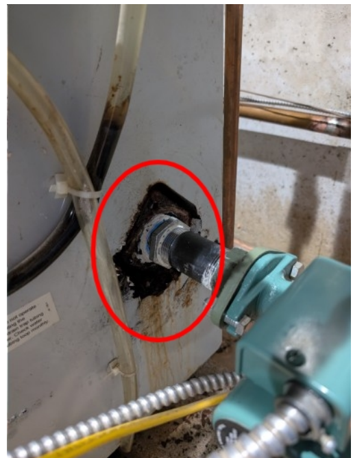
Corroded Section of Boiler
